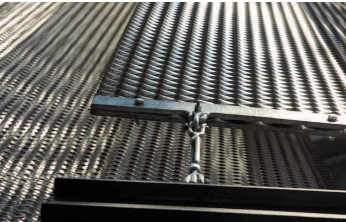
Anchoring of the strip at the bottom.
